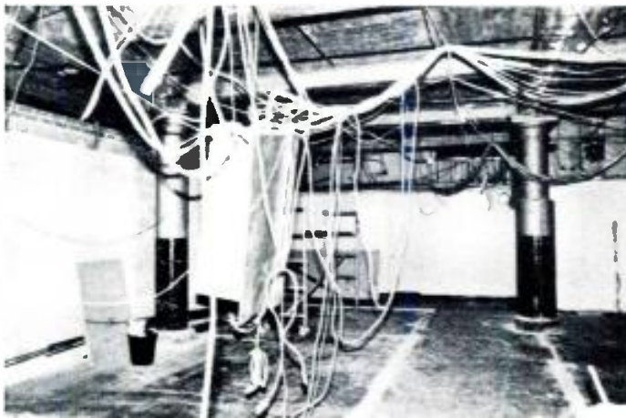
Roughsite after demolition showing main building columns and phone junction box.
