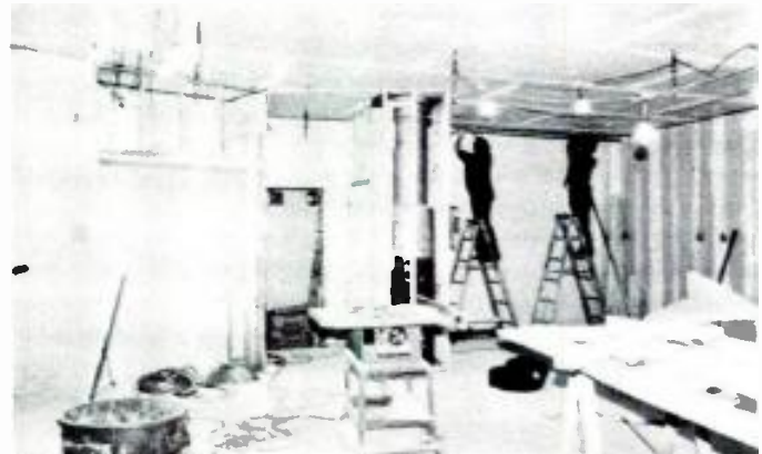
Rear of room showing framing of 15-foot semi-circular couch, sound trap panels suspended in cavity behind.
